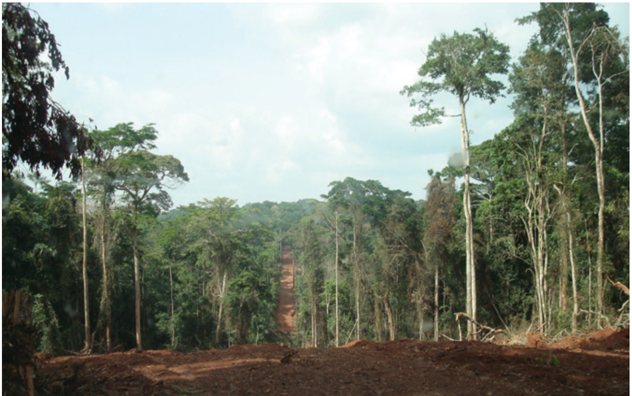
Initial clearing for Tailings Dam site
